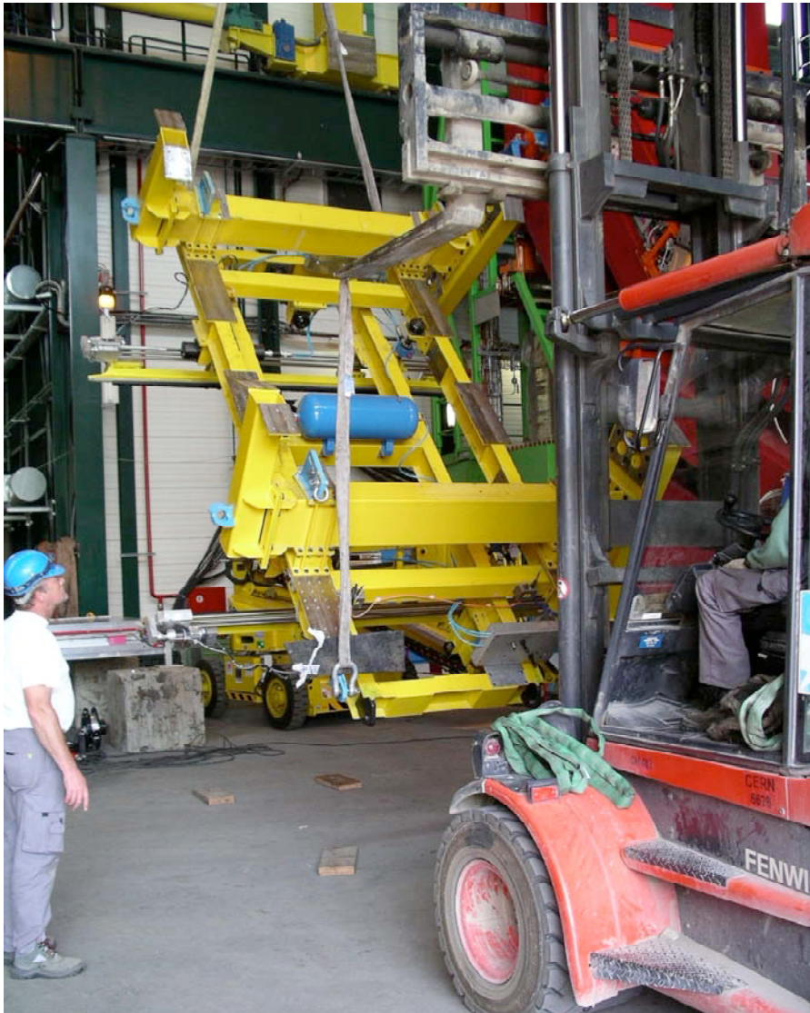
Cradle rotation with forklift
