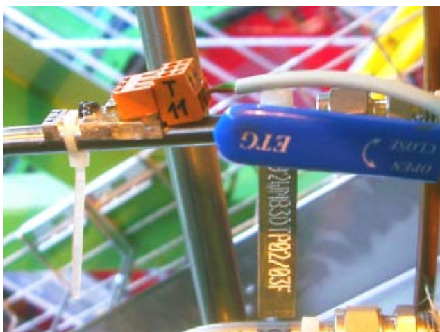
Sensor at supply line of distributor.
