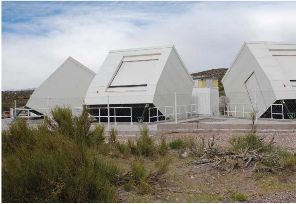
Figure 4.13: A picture of the three tilted HEAT telescopes. Behind the middle telescope the DAQ container, which houses the shared electronics for all HEAT telescopes is visible. Further in the back a part of the standard fluorescence building Coihueco is visible. Picture source: H.O. Klages, KIT
