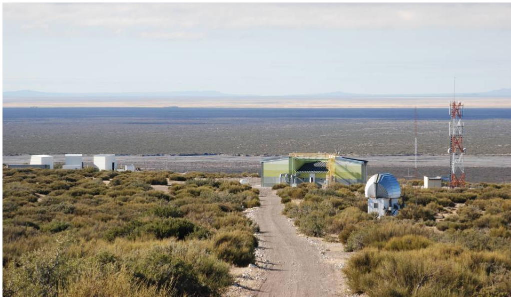
Figure 4.14: View over part of the infill array from behind Coihueco and HEAT. On the left side the three HEAT telescope shelters in downward mode are visible. The green building on the right is the standard FD building Coihueco. On the right side of Coihueco the radio communication tower is visible. The structure with the metallic dome in front of Coihueco is a LIDAR, a part of the atmospheric monitoring of the observatory.
