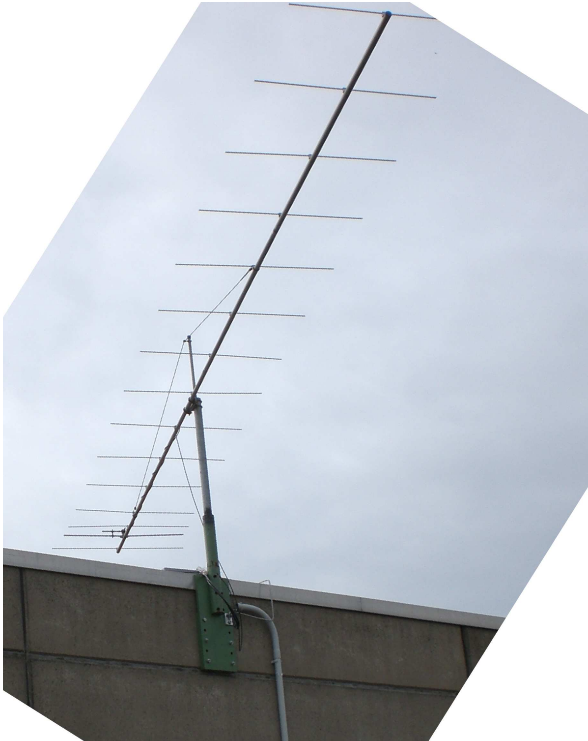
Figure 29: Picture of the 2 m band antenna mounted on top of the Physikzentrum in Aachen.
