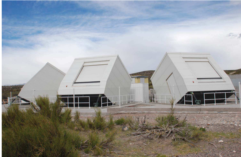
Figure 3.7: Photo of the 3 tilted HEAT bays [74].
