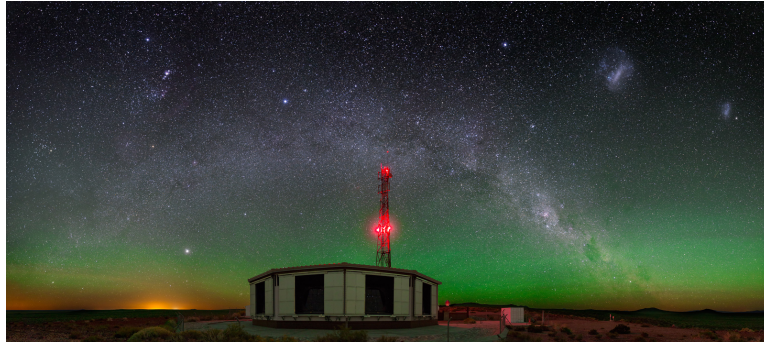
(a) Fluorescence telescope building (Los Morados). Each building contains six telescopes and is accompanied by a tall communication antenna.
