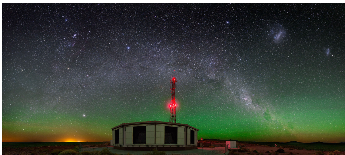
Figure 3.4: Areal photo including a fluorescence telescope building (Los Morados) of the fluorescence detector of the Pierre Auger Observatory. Each building contains six telescopes and is accompanied by a large communications antenna. Photo courtesy of S.Šaffi.
