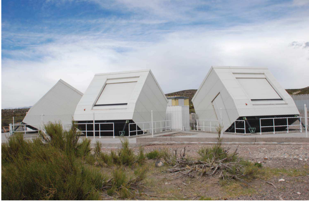
Figure 6: Photo of the HEATs tilted in "upward" mode [4].
