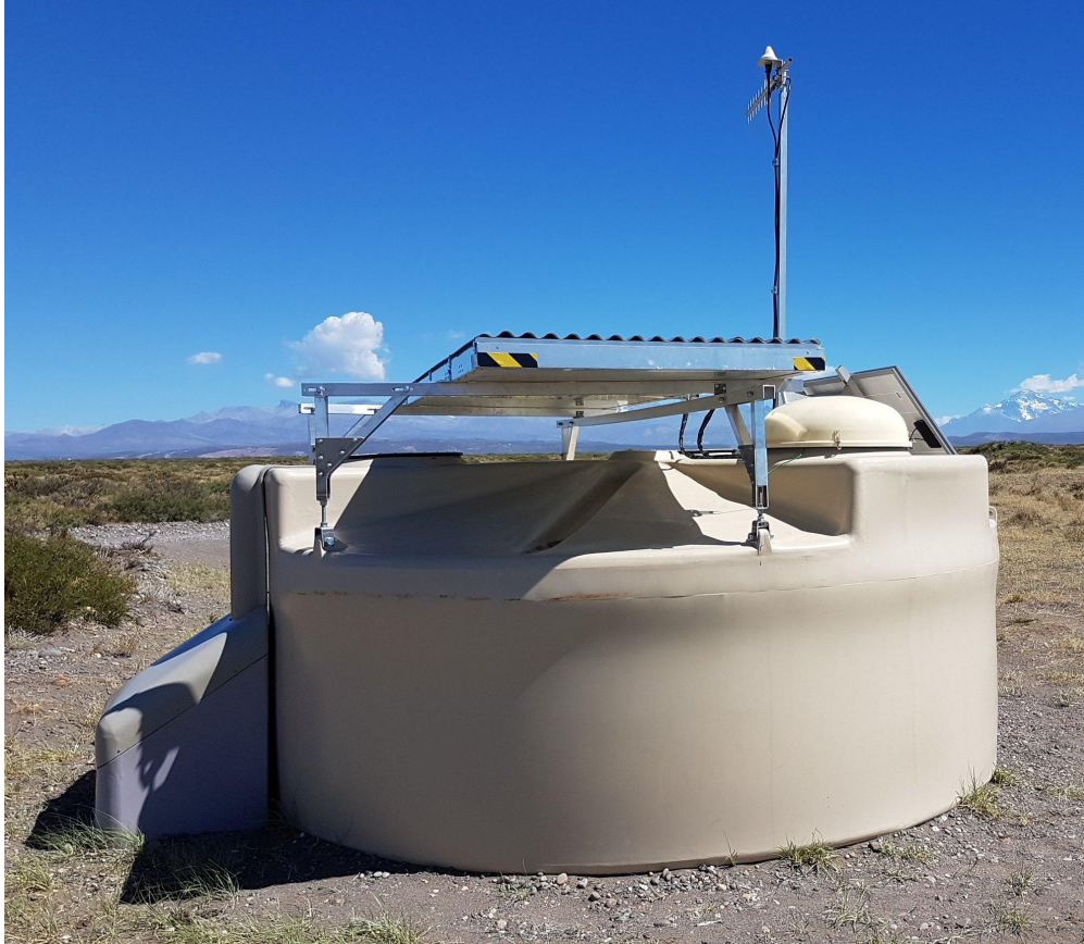
Figure 3.10. Field photo of an SD station where an SSD has been installed over the WCD [160].
