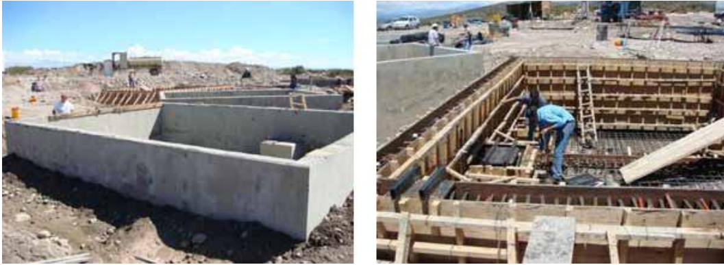
Figure 19: Foundations of the three HEAT telescopes.
